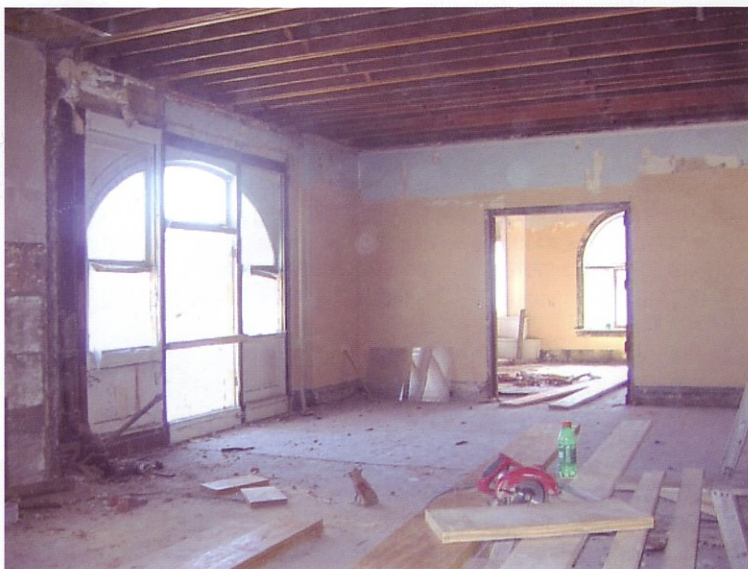
Interior Walls Removed - Looking South Towards "Founders Room"
